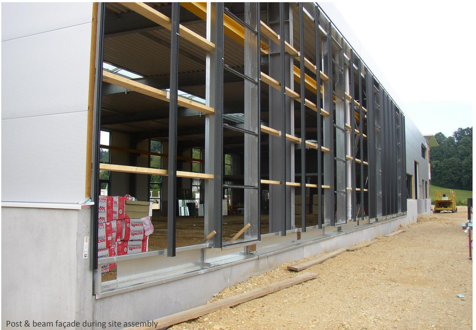
Energy façade – Thermal and daylight elements arranged alternately
